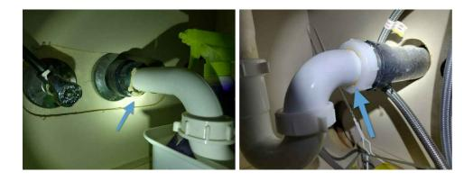
7.8.2 Sinks & Faucets CALCIUM/CORROSION AT SUPPLY VALVES KITCHEN AND BOTH BATHROOMS
