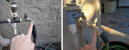
7.7.2 Exterior Hose Bibs **LEAKING HANDLE(S)**
