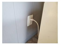
8.6.5 Receptacles & GFCI Devices **DAMAGED RECEPTACLE/COVER**
