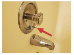
7.10.1 Toilets CALCIUM/CORROSION AT SUPPLY VALVES GUEST BATHROOM
